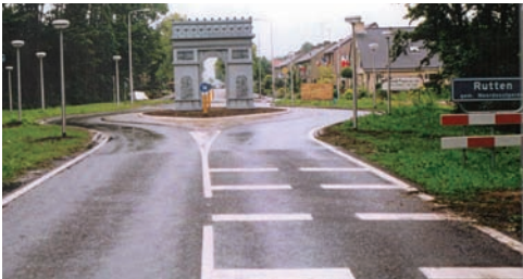
Area boundary on distributor road, with a large central island
