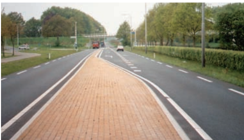
Priority intersection outside the built-up area with narrow traffic island and left-turn lane
