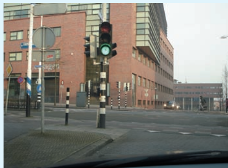
Photo 13.3. Arrow sign is too far to the left
