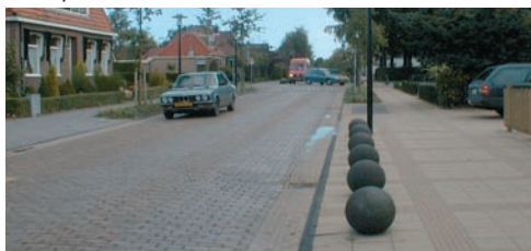
AR-30, access roads
