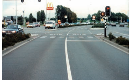
Bus lane, central position with intersection with traffic light control system (Eindhoven)
