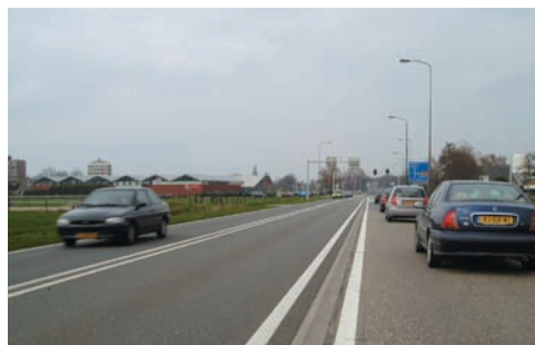
Distributor road, raised bus lane, centrally positioned, tidal flow with lane control signing
