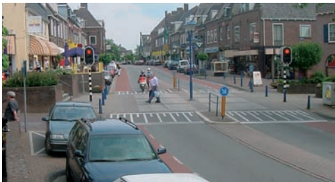
Crossing on a distributor road with a raised section and traffic light control system (separation in time)
