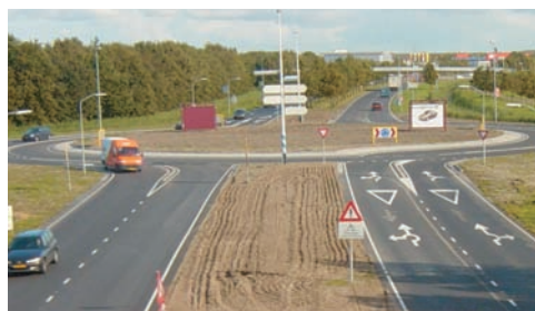
Multi-lane (turbo) roundabout (outside the built-up area)
