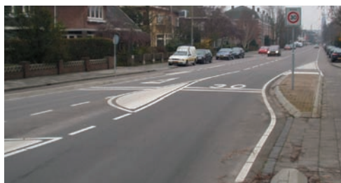
Grey road, major discrepancy between the intended access function and the design
