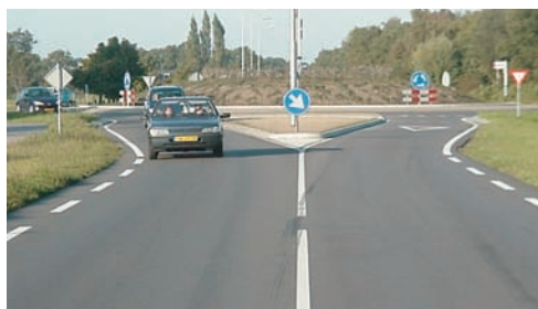
Roundabout with single lane entry and exit road
