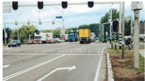
Priority intersection with traffic light control system, raised road section and red light and speed camera
