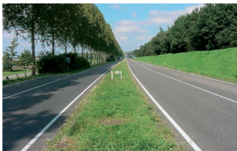
Distributor road, bus lane on right
