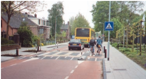
Crossing (raised section) at the entrance
