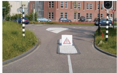
Barrier, road open to public transport buses only
