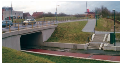
Grade-separated solution near a bus stop in combination with a bicycle path
